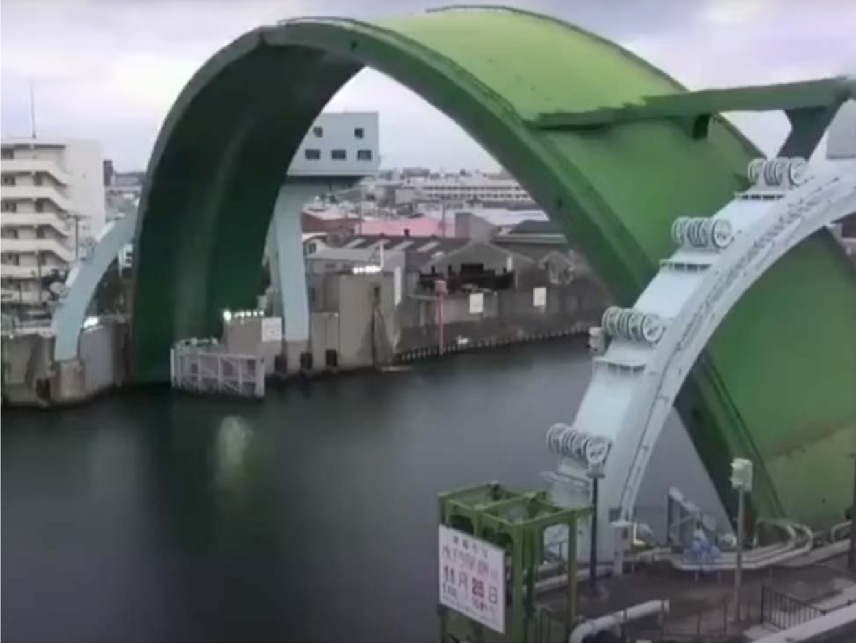
protect from typhoons and storm surges in Osaka, Japan.
